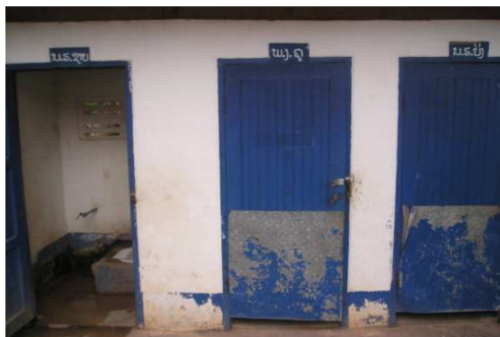
Figure 4.10: Typical sanitation facilities in a school
